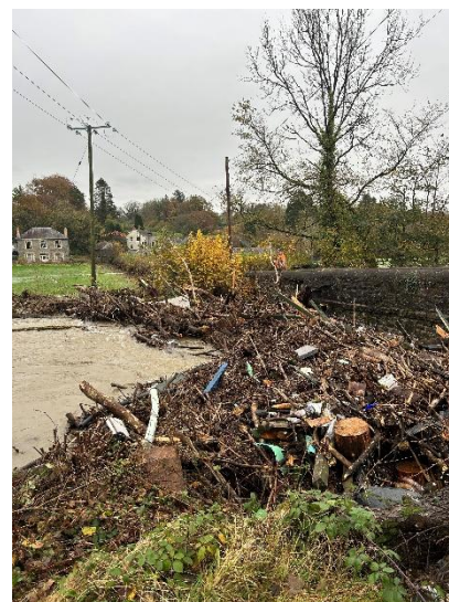
Flooding and debris blocking bridge in Brownnydd, Carmarthen
